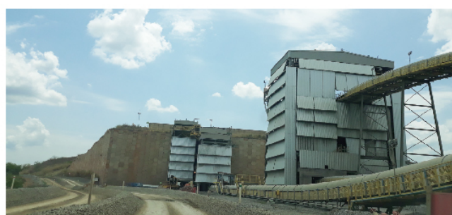
The enclosure of the crushing system of Boa Vista Mine was carried out in order to minimize the noise of the operation and minimize the emission of particulates to the atmosphere.
