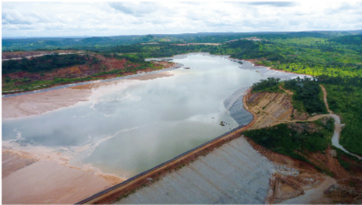
▲ Tailings produced by our TFM copper and cobalt mine in the DRC are currently being deposited in a TSF with a total storage capacity of 66 Mt. A new TSF is currently undergoing construction adjacent to the first, which will bring the cumulative storage capacity to 147 Mt. Current estimates of the life of mine for our oxide deposits at this property indicate that additional storage capacity will be necessary to accommodate future production of tailings beyond this current expansion. The TSF at TFM is fully lined so as to protect groundwater resources of importance to our communities.
