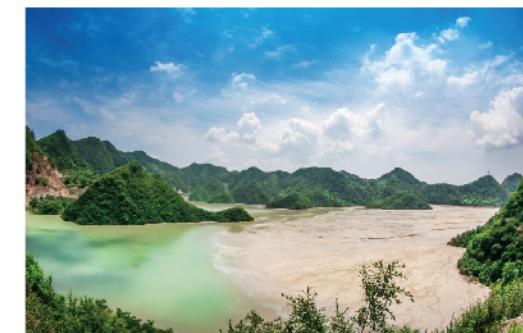
▲ In China, the water we use for production is fully recycled after sedimentation in the tailing ponds, so only a small amount of river water would be used as supplement. Waste water produced during ore selection is shipped to the tailing ponds using sand pump and becomes recycled clean water after being diluted and clarified there. Then 100% of the recycled clean water would be re-pumped to the closed water circuit. Water we used for cleaning the operation equipment are all recycled clean water, which are pumped to designated taps for flushing equipment and manufacturing sites. The water used after flushing would be drained to the emergency pool for the discharging plant or the tailing pools located within the factory through drains and gutters. Those waste waters collected in the discharging plant would be pumped through sand pumps to thickening pool, from where it would be sent to the tailings pond using reciprocating pumps.
