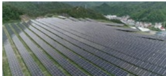
At our Chinese operations, we have installed photovoltaic power stations at retired tailings storage facilities.
